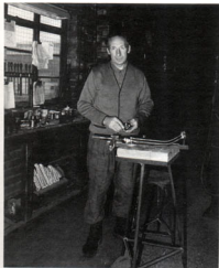
Figure 8-3: Norman Taylor in his workshop with the simple Taylor-design fork jig.
